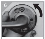
• Rotate rose furniture to align screws with countersunk holes.
